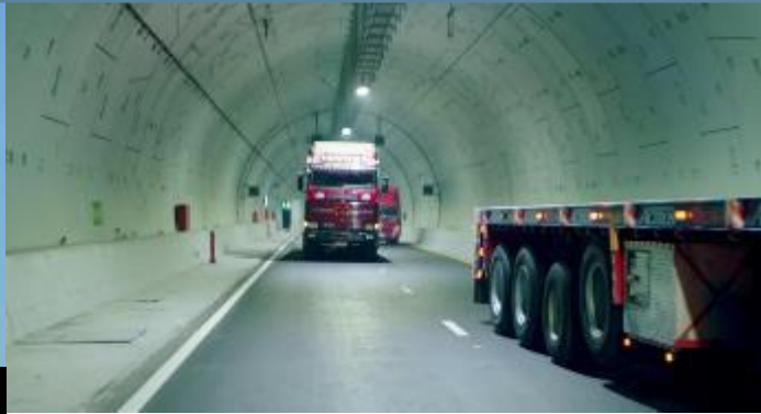
EPS PORT Roads & Tunnels
